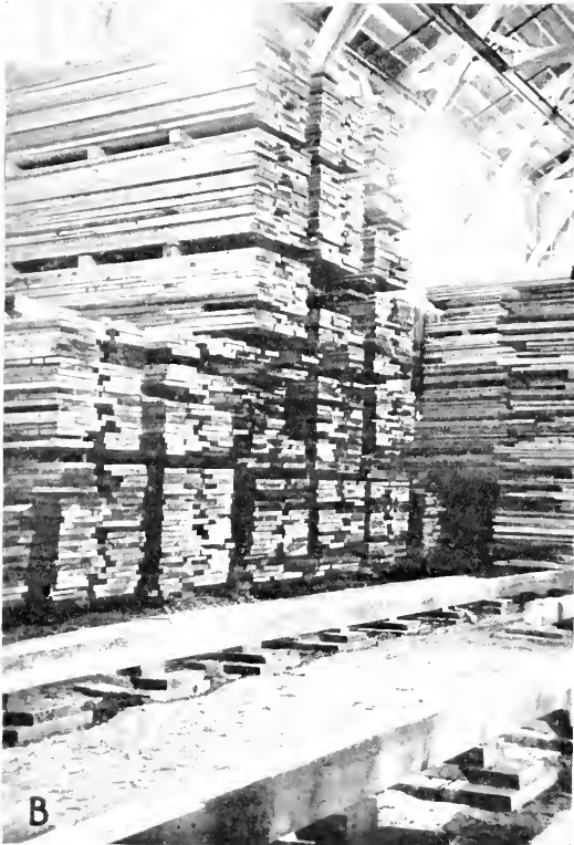
Storage of seasoned lumber under shelter: A, The exterior of a storage shed suitable for air-seasoned lumber, showing its one open side; B, a part of the interior of the same well-built shed. The lumber is bulk piled flat on stringers, with heavy stickers separating successive piles; additional stringers at the ends of the piles might be better practice than the small number now used
